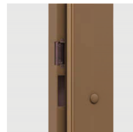
adjustable strike - steel door frame (optionally)
